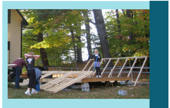
Team members building storage shed
